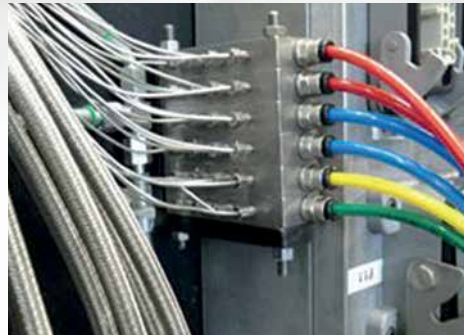
Pose de tubes inox 2
